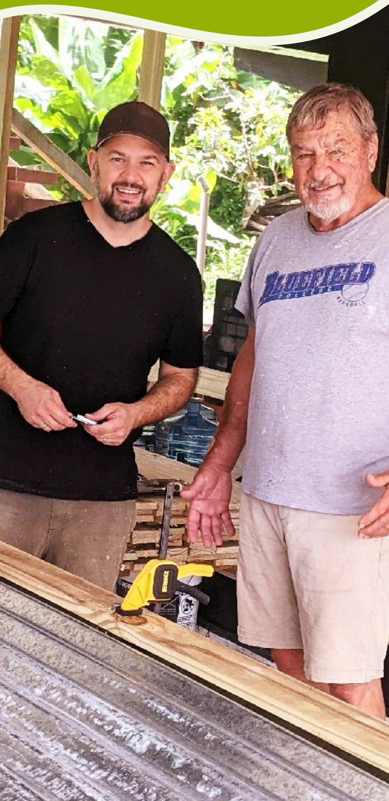
PHOTO: DAN AND HENRY (A GUEST) BUILDING MOBILE WALLS
